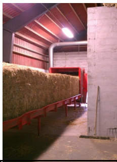
Straw for heat- Straw bales being conveyed into a combustion heating system for a 26 building farm estate
